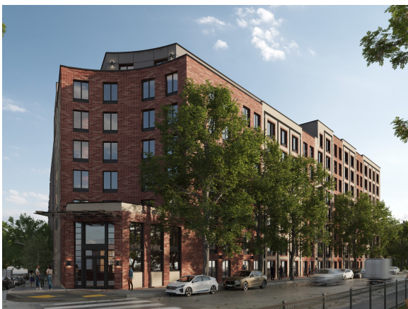
Developed by Tishman Speyer , 160 Van Cortlandt Park South is an eight-story, 339-unit affordable housing project underway in the Bronx's Kingsbridge neighborhood. The building is being constructed to Enterprise Green Community sustainability standards. Image by Aufgang Architects , courtesy of Tishman Speyer
